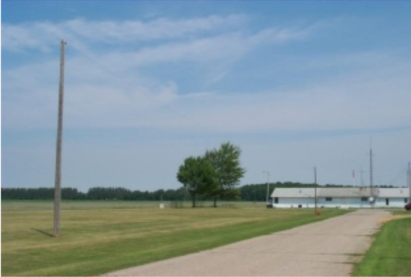
Our next stop was Three Rivers, Michigan - the home of powerhouse **HAI** on 407 kHz. Three Rivers is also in Saint Joseph County and is about twenty minutes from Sturgis on state highway M-60, via US 12 and US 131. The Three Rivers airport is on M-60 just east of town. The NDB is in the MHW class and is about as plain as they come with two telephone poles
